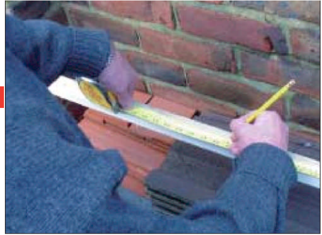
- Right handed people tend to hold a tape in their left hand and mark off with the right. This results in the numbers on the tape being upside down.
