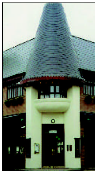
- Forming a truncated half cone in double lap slates can be achieved with planning and quality workmanship. (Photo: Red Bank Manufacturing)
